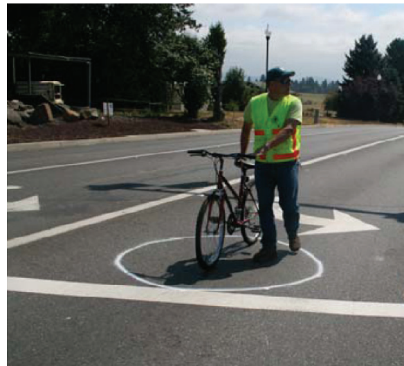
Bicycle Loop Detectors Can be Designed for Traffic Signals
